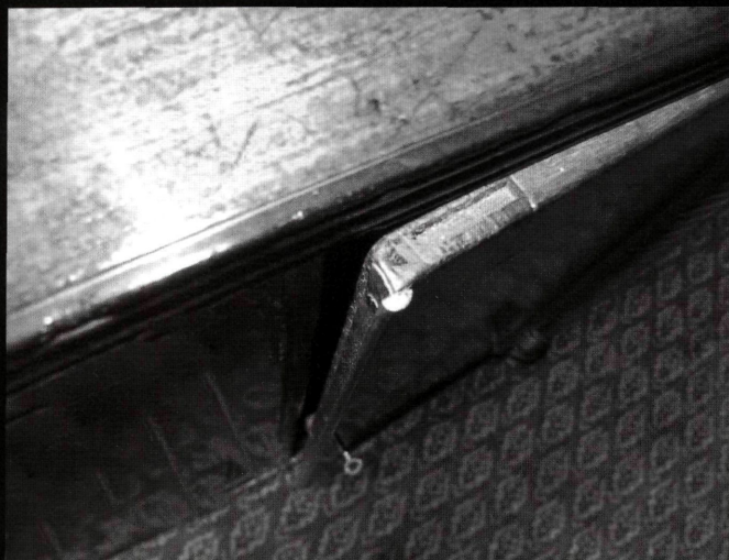
Plate 6. Detail of lead filled astragal bar
