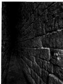
Plate 4. *Clyde Bank*, the original unrendered northern brick wall. Restricted access between the two buildings has made the complete rendering of this wall impossible.
