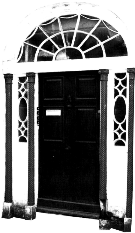
Plate 10. This doorway in Main Street, Kinsale, Co. Cork provides a contemporary, immovable source of this form of decoration in carved wood, the house c. 1810.
